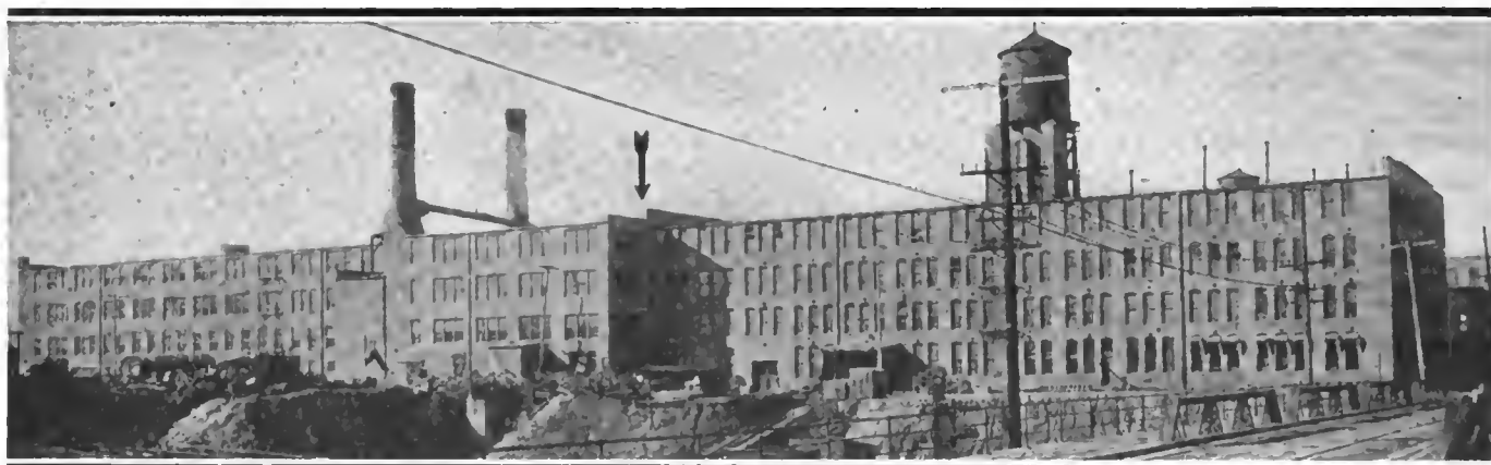
Plant of the Racine Mfg. Co., Racine, Wis., the portion to the left of the arrow being the large addition made this year. The additional floor space amounts to 200,000 square feet. Cost of additions was $75,000
